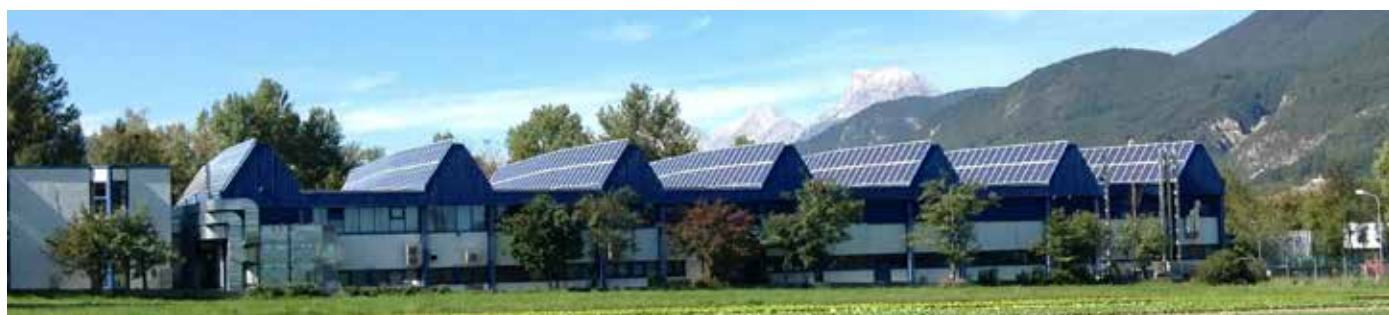
Sustainability orientated production: e.g. use of solar energy in Kematen, Austria
